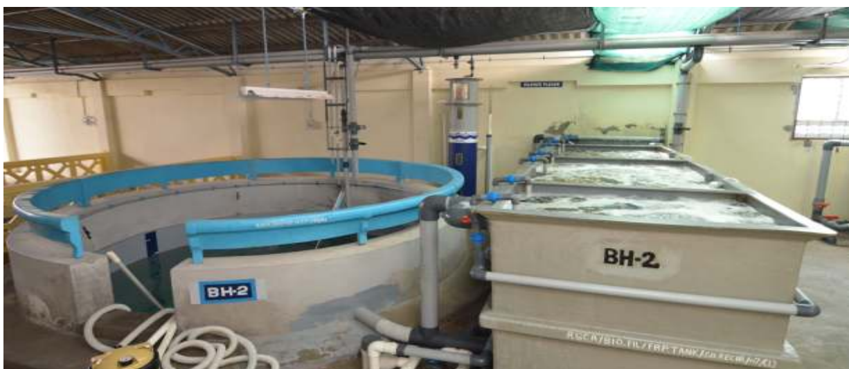
Bio filtration systems for Seabass brood stocks
